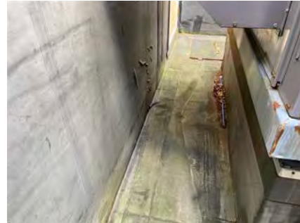
Image 2 – Monitor Well EPDM roof and walls.
