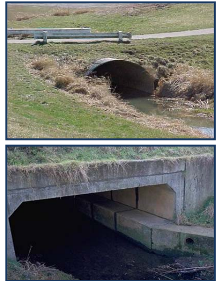
Before Mitigation and After Mitigation
