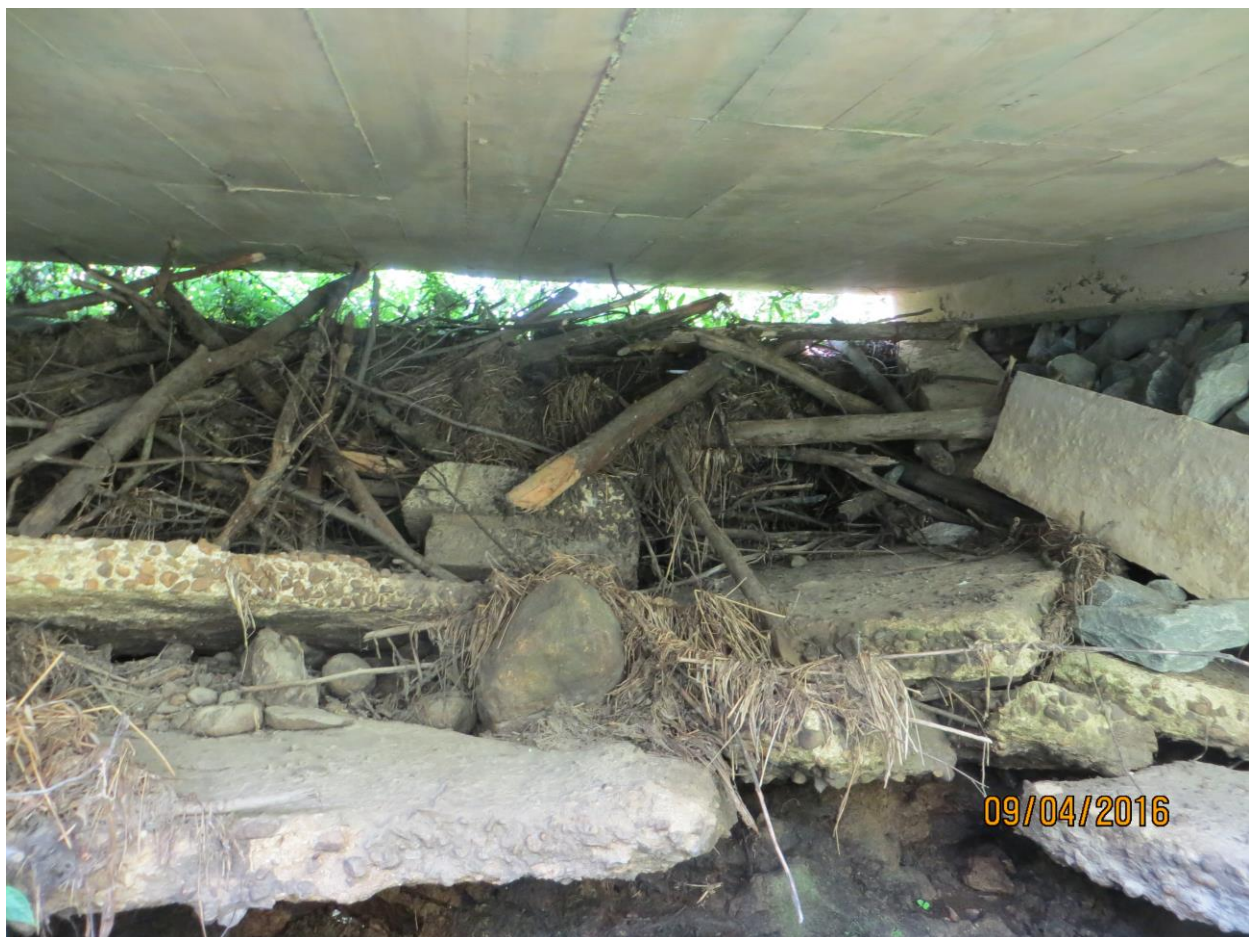
Underside of Spillway #1.
